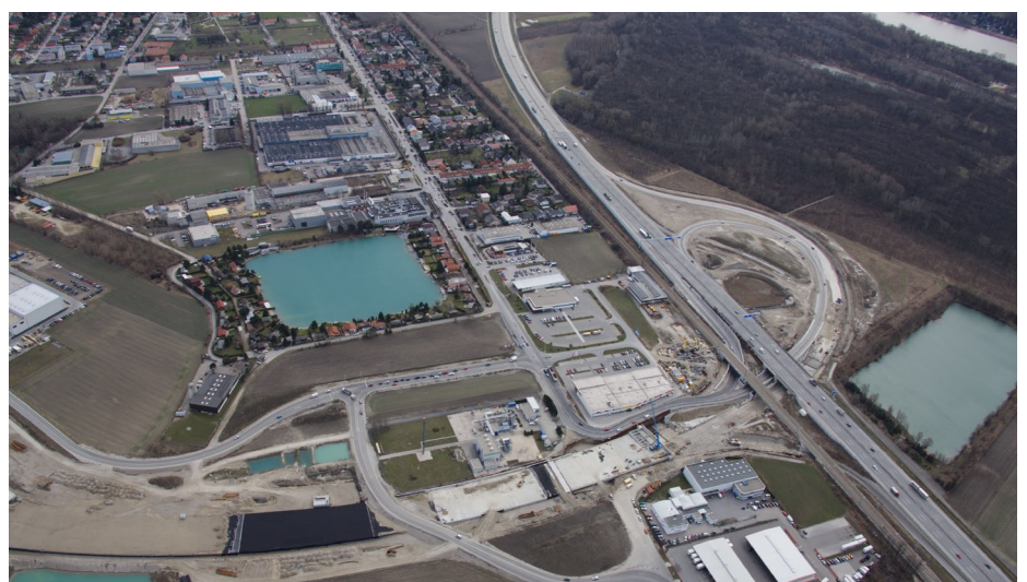
Aerial view of Kreuzenstein Tunnel
