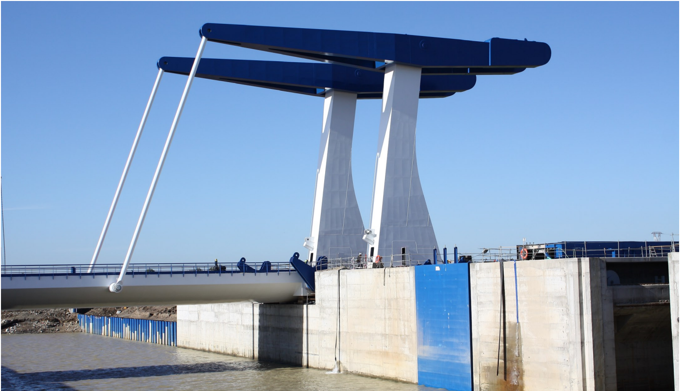
Drawbridge over the lock's navigable channel
